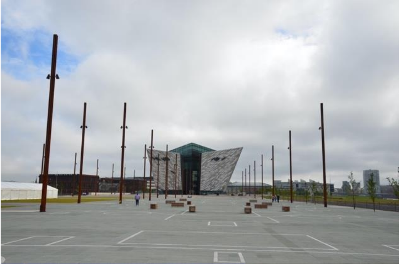
This is the shipyard where Titanic was built. Looking towards Museum.
